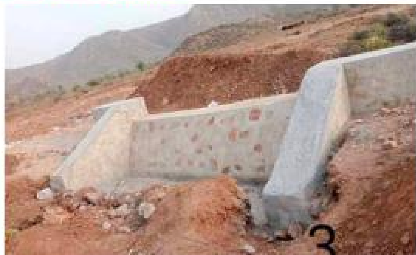
One of the completed Small Water Harvesting Structure at Alwar, Rajasthan
